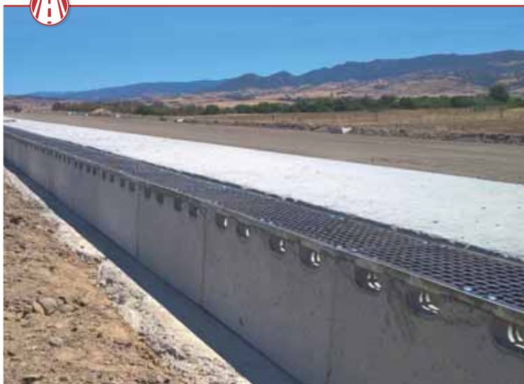
National Road S.S. Sassari - Olbia Drainage channels (Sardinia, Italy)
